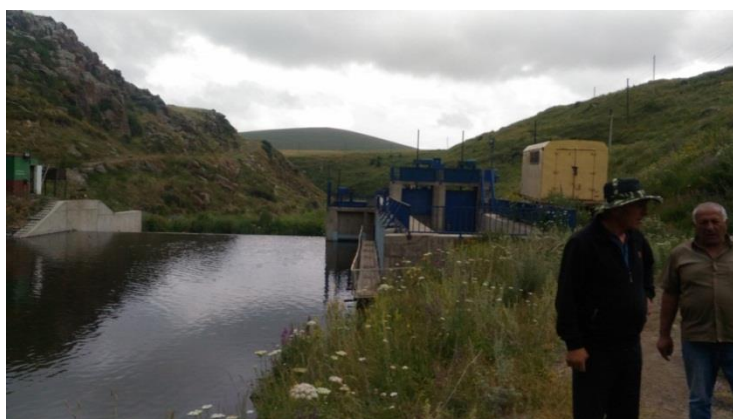
Figure 17: Vardenik SHPP (Water Abstraction Structure) (2018)
