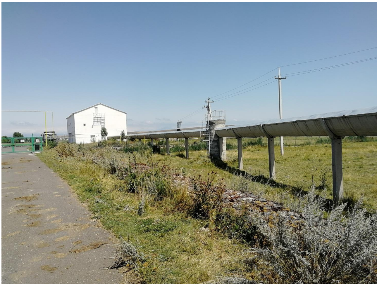
Wastewater Treatment Plant in Artsvakar District of Gavar Town
