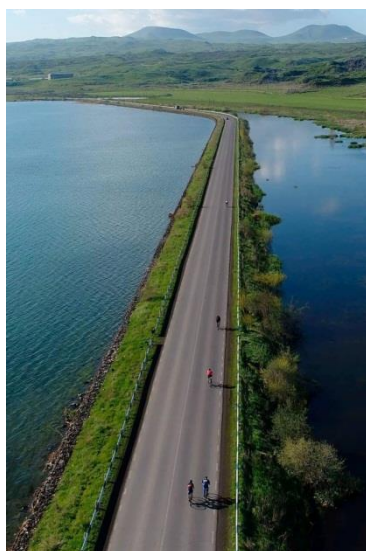
Figure 21: M10 Inter-State Road near Lchashen Village (2017)
